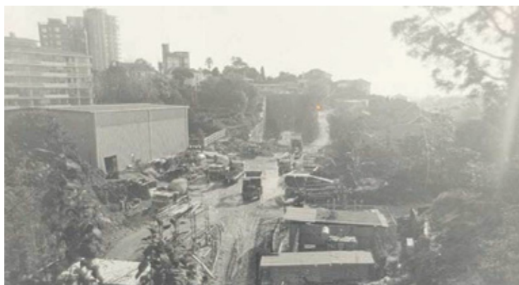
Work well underway on the cutting and proposed Woollahra Railway station, visible from Wallaroy Road in the 1970s. Photograph courtesy Woollahra Libraries
